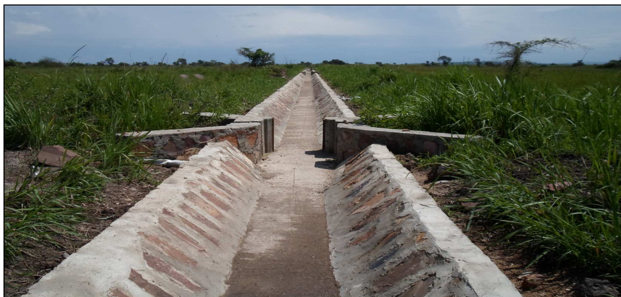
Irrigation Infrastructures at Kyakakera –Kashaba
